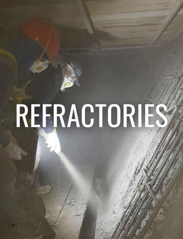
With more than a half century of installations, our chemical-resistant refractories are well known for their thermal insulating characteristics and speed of application. This material is resistant to high acid concentrations and temperatures up to 2100°F.
