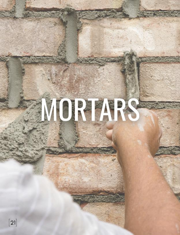
Sauereisen's extensive selection of mortars range from silicate mortars for high acid/high temperature environments to organic mortars for broad chemical resistance. Typical installations are completed by either the brick layer's or tile setter's method of application.
